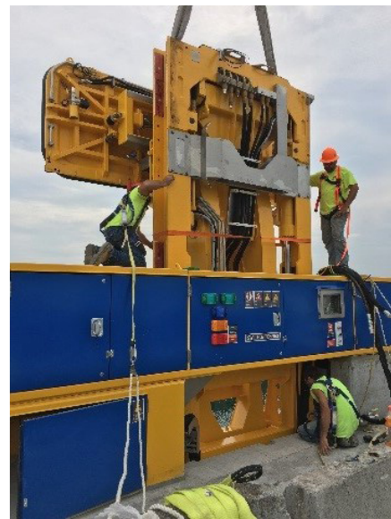
View From Lock Wall: HFM dynamic head unit with vacuum pads being lowered into position at Eisenhower Lock.
