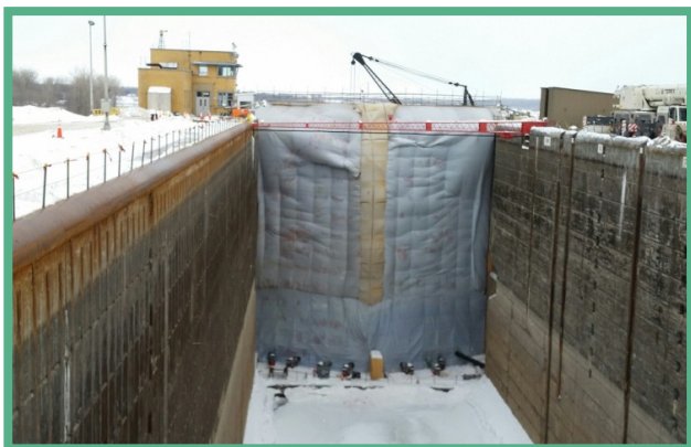
Blast cleaning and painting miter gates at Snell Lock in Massena, N.Y.
