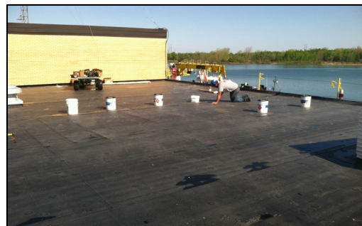
Workers install a new EPDM roofing system at the SLSDC's maintenance facility in Massena, N.Y.
