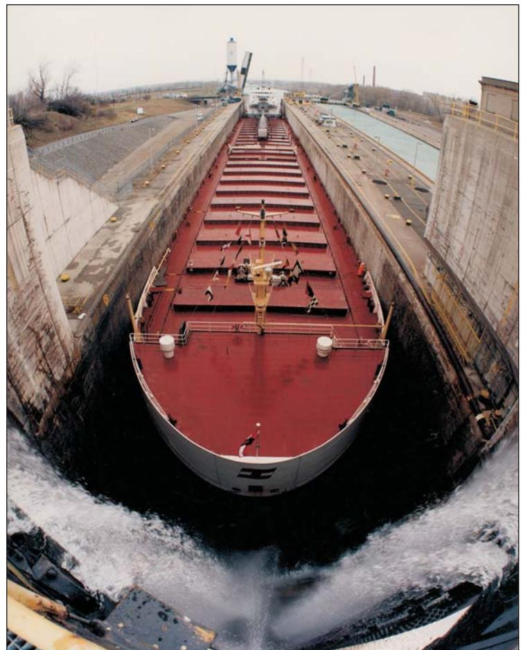
Vessel being raised in a lock
