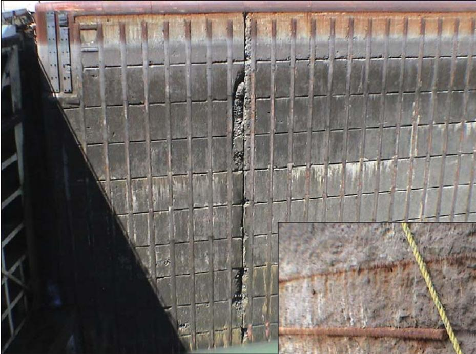
North Lock Wall at Snell with Vertical Wall Armor. (Note typical damage at monolith vertical joints)
