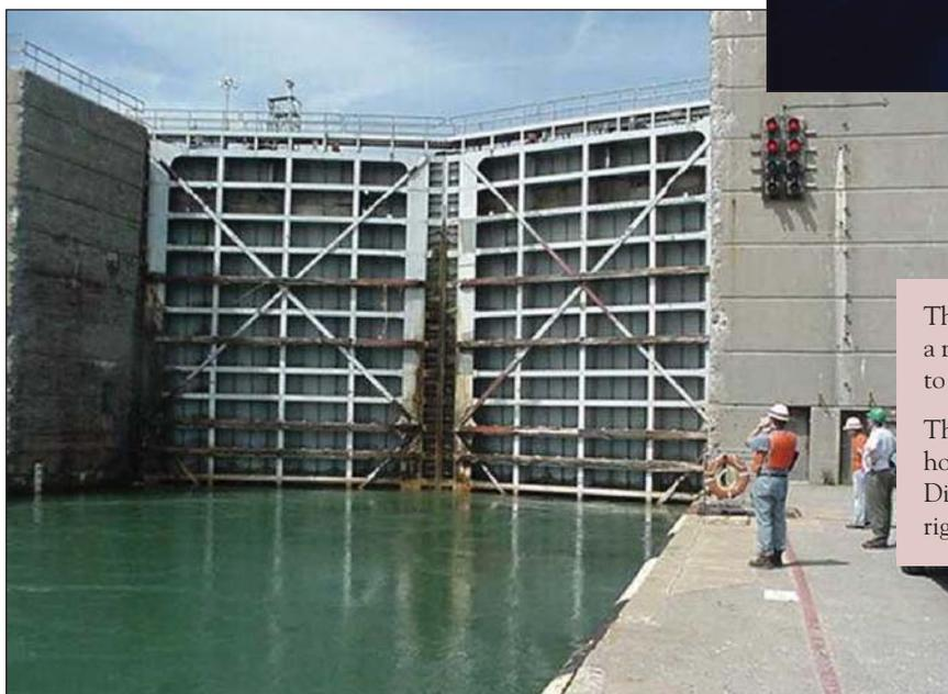
This massive gate must be capable of maintaining a nearly water-tight seal. At the same time it needs to be opened and closed on a routine basis.
